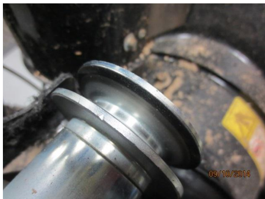
Before polishing – rough surface near top of pulley
